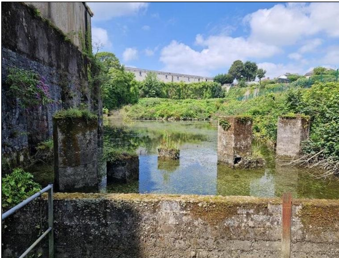
Figure 11-15 Reservoir with concrete piers designated for removal.
